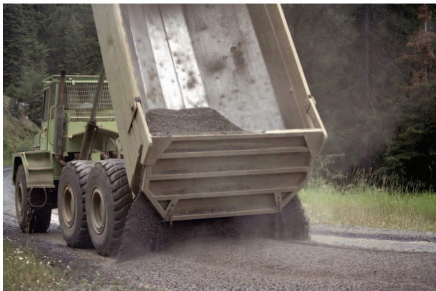
Roads on working forestlands are being repaired and maintained to prevent sediment from entering streams. Photo by Keith W. Wood, courtesy the Washington Forest Protection Association.
