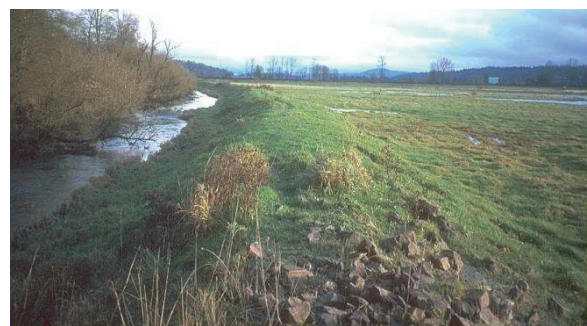
Cherry Creek, King County. Dikes separate rivers from their historic side channels, wetlands, and floodplains. Photo courtesy the Washington State Salmon Recovery Funding Board.
