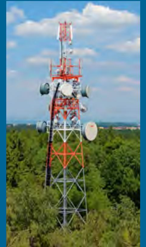
The eight DTV/HDFM stations are connected by **12 microwave radio** sites covering more than **550 miles**. Each microwave site has a tower in the **300-foot range** with lighting at night to be visible to aircraft.
